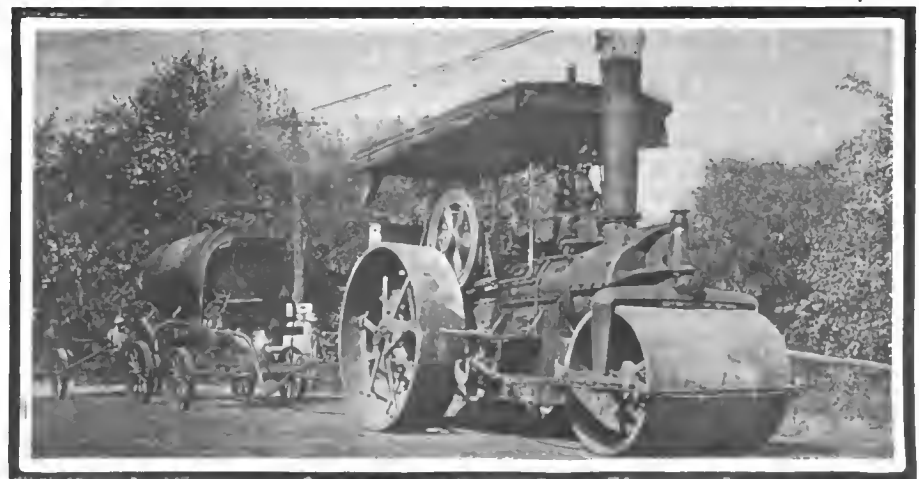
Tractor roller, drawing hot oil tank and pressure oil-spraying machine
